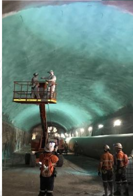
Waterproof membrane being applied in NorthConnex tunnel
