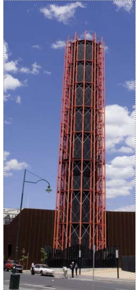
^ CityLink ventilation stack.
