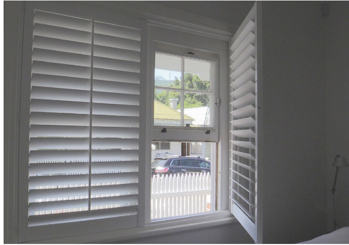
Figure 9: The open window and louvered shutters at M's house less than 50 metres from the sound wall.
