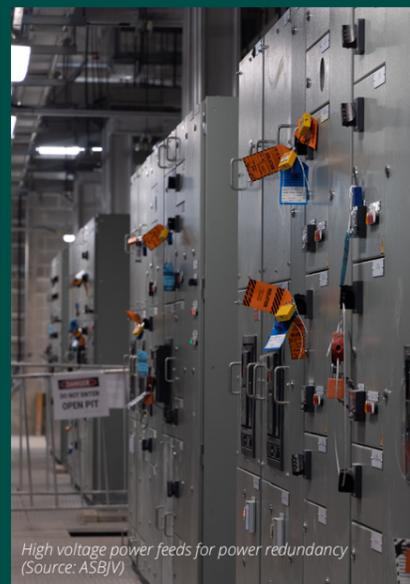
High voltage power feeds for power redundancy (Source: ASBJV)
