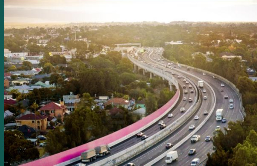
Completed M4 widening – Stage 1A of WestConnex
