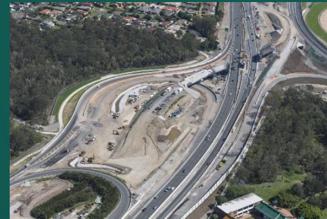
Gateway Upgrade North construction continues
